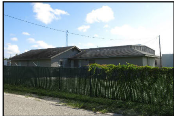
Photo 5.9. 2522 Hunt Road (8PA02112), looking northeast.
