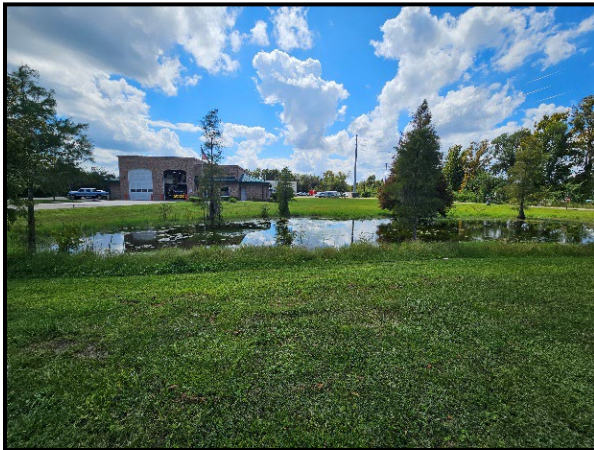
Photo 2.21. View of fire station and existing pond within north and east portions of Pond C(1), facing south.
