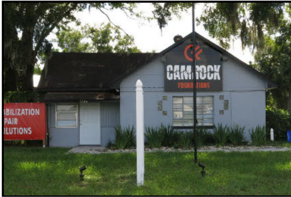
Photo 5.6. 2514 U.S. Highway 41 (8PA01498), looking east.
