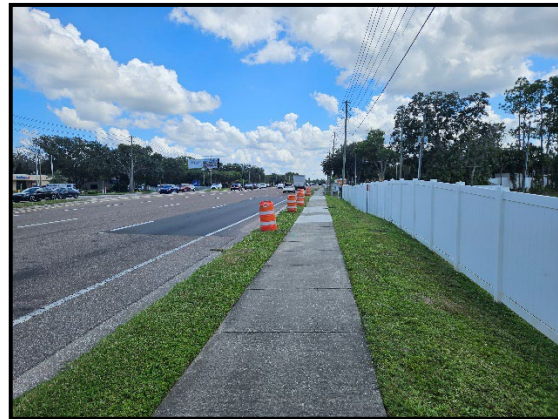
Photo 2.6. View of south side of east corridor of SR 54, facing east.
