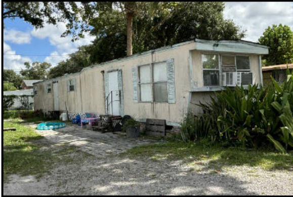
Photo 5.31. 21307 McKaig Lane (8PA03796), looking northeast.
