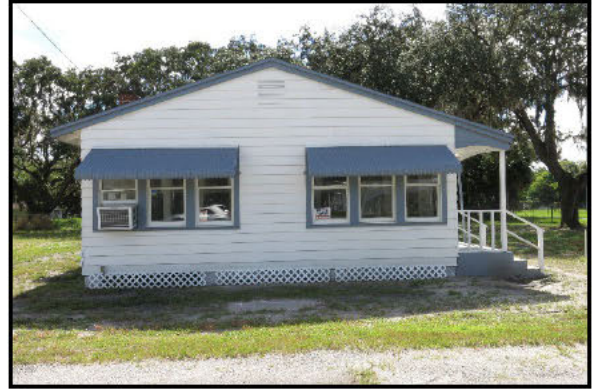
Photo 5.23. 2720 U.S. Highway 41 (8PA01499), looking east.
