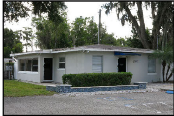
Photo 5.7. 2810 U.S. Highway 41 (8PA01500), looking southeast.
