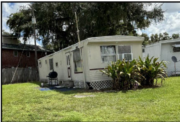
Photo 5.37. 21301 Rustic Lodge Lane (8PA03802), looking northeast.
