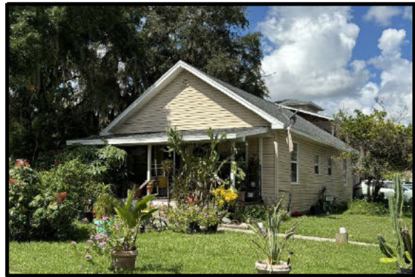
Photo 5.25. 21324-21326 Paoli Drive (8PA02832), looking southwest.
