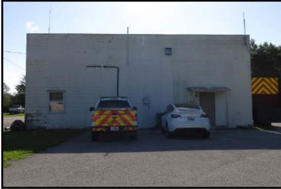
Photo 5.14. 21300 State Road 54 (8PA03789), looking east.
