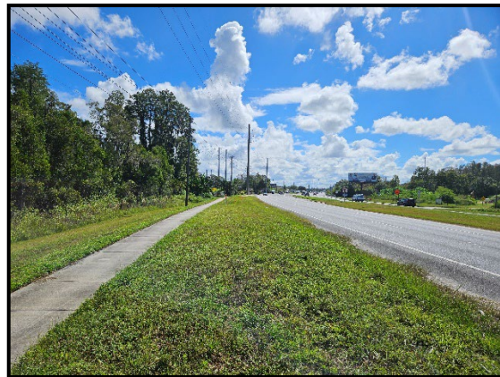
Photo 2.2. View of environment and utilities in the western corridor along north side of SR 54, facing east-southeast.
