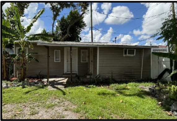
Photo 5.24. 2836 U.S. Highway 41 (8PA01501), looking south.
