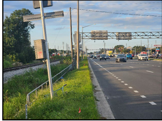
Photo 2.10. View of drainage/utilities along west side of south US 41 corridor adjacent Seaboard Coastline Railroad, facing north.
