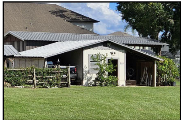
Photo 5.38. 20430 SR 54 (Outbuilding 1) (8PA03808), looking east.
