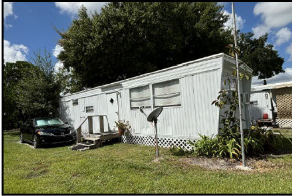
Photo 5.35. 21308 Rustic Lodge Lane (8PA03800), looking southwest.
