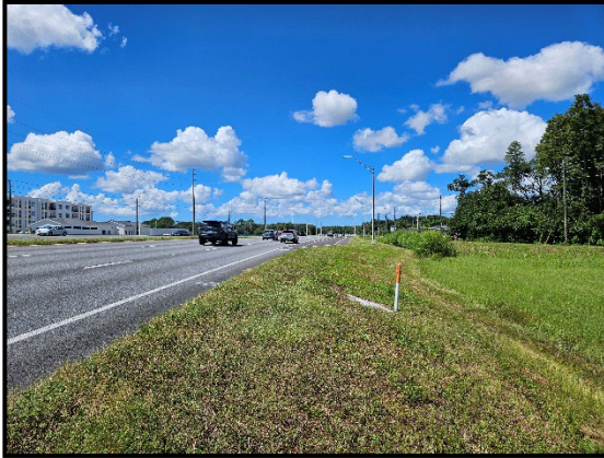
Photo 2.3. View of drainage and utilities along north side of SR 54 toward west end of the west corridor, facing west.
