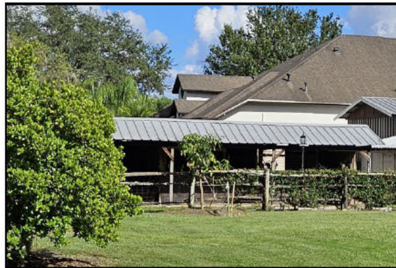
Photo 5.39. 20430 SR 54 (Outbuilding 2) (8PA03809), looking east.
