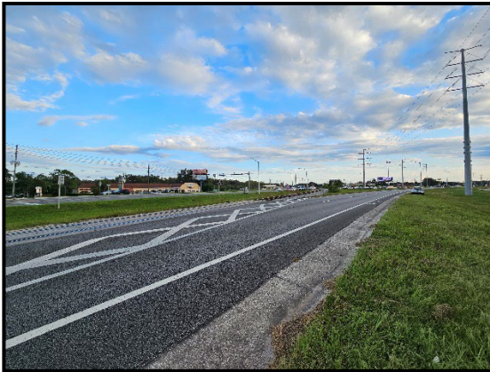
Photo 2.11. View of Land O'Lakes/Dale Mabry Highway interchange in south corridor from west side, facing southeast.
