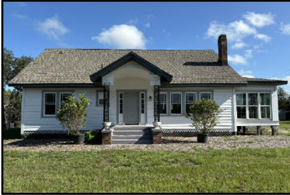
Photo 5.22. 2515 Hunt Road (8PA00303), looking north.
