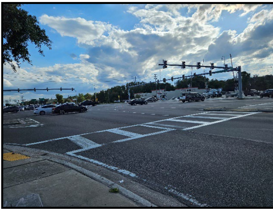
Photo 2.1. View of US 41/SR 54 intersection from the northeast corner, facing southwest.
