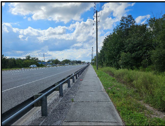
Photo 2.7. View of guardrail, sidewalk, and drainage ditch along north side of east SR 54 corridor, facing west.
