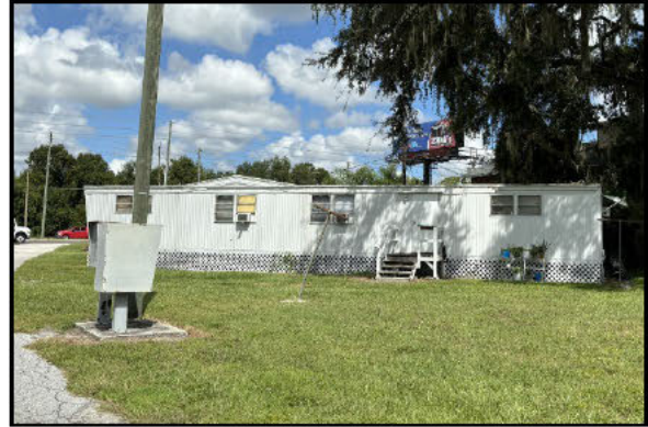
Photo 5.36. 21303 Rustic Lodge Lane (8PA03801), looking northeast.
