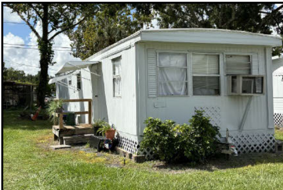
Photo 5.33. 21304 Rustic Lodge Lane (8PA03798), looking south.
